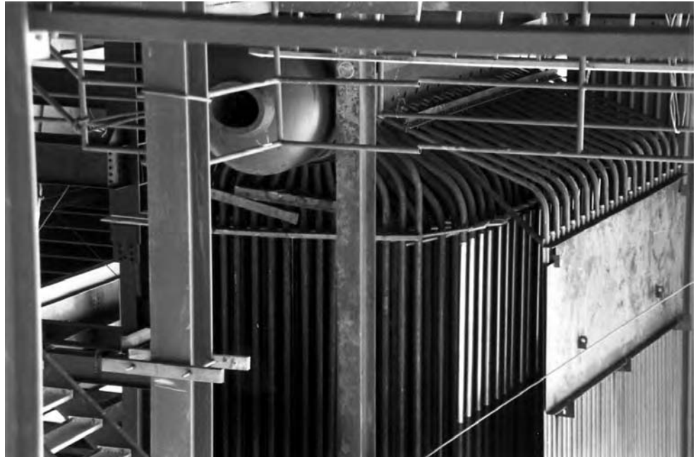
Figure 7-9 Boiler tubes for steam generation. (Courtesy P. Aarne Vesilind)
