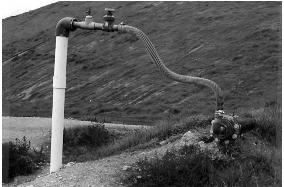
Figure 4-21 Gas extraction well in place. (Courtesy William A. Worrell)
