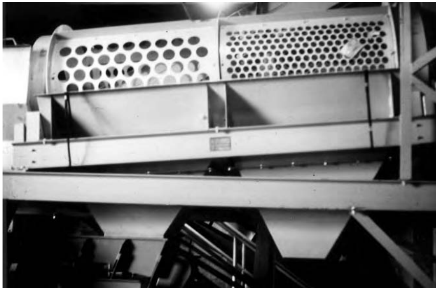
Figure 6-4 Trommel screen. (Courtesy P. Aarne Vesilind)
