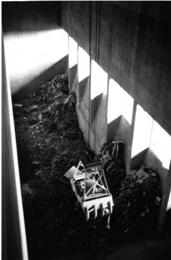
Figure 7-7 Storage pit and crane in a typical MSW combustor. (Courtesy P. Aarne Vesilind)
