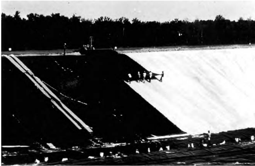
Figure 1-9 Placement of a synthetic liner in a modern landfill. (Courtesy P. Aarne Vesilind)
