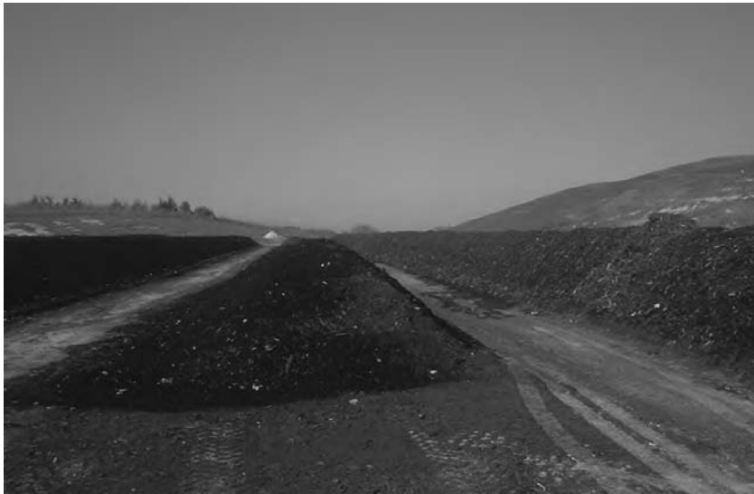
Figure 8-4 Windrow composting system. (Courtesy William A. Worrell)
