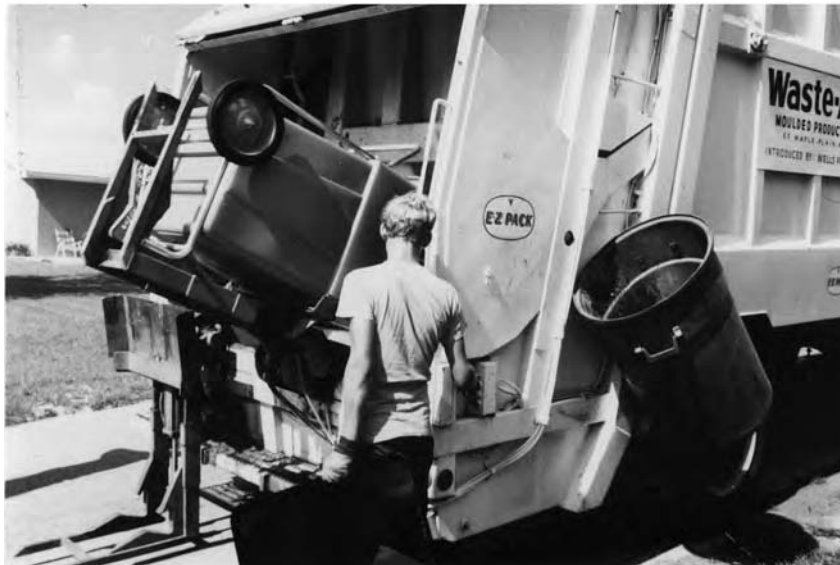
Figure 3-6 Green plastic containers used for solid waste collection. (Courtesy P. Arne Vesilind)
