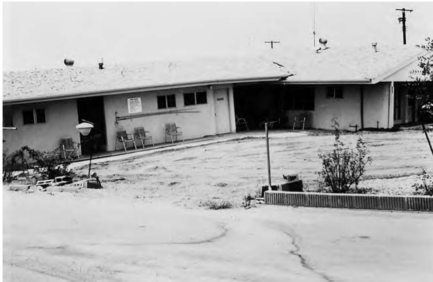
Figure 4-22 An unfortunate motel built on a settling landfill. (Courtesy P. Aarne Vesilind)
